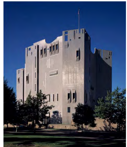
The Denver Art Museum’s iconic 1971 North Building, designed by Gio Ponti and James Sudler Architects of Denver.
