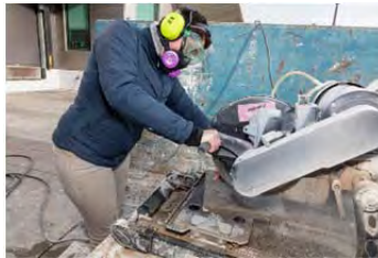
Daisy Quezada installing Desplazamiento/Contención (Displacement/Containment) . Photo by Jeff Wells. Courtesy of the artist and the Denver Art Museum.
